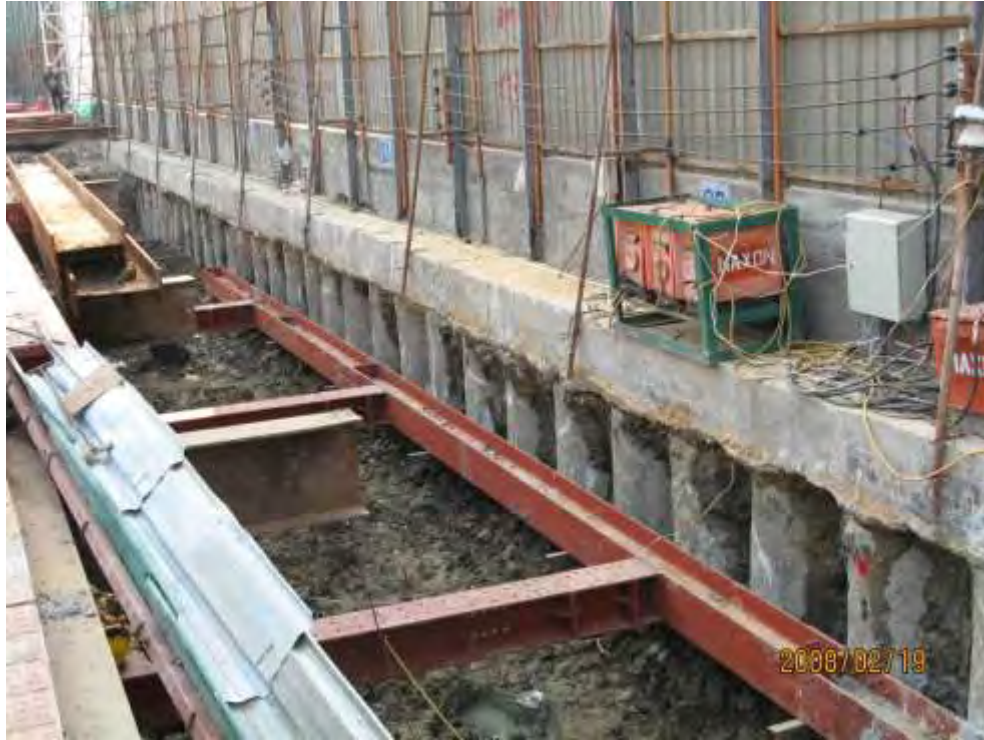
Figure 7. Photograph of pile wall construction
