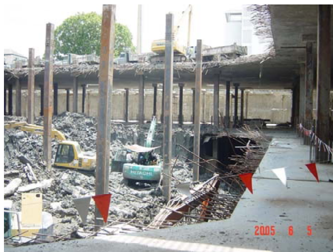
Figure 17. Photograph of excavated soil at opening area
