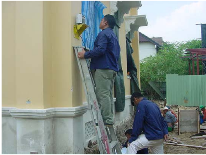
Figure 7(a). Photograph of tiltmeter measuring at Tewavej palace
