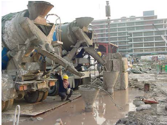
Figure 15. Photograph concreting of diaphragm wall
