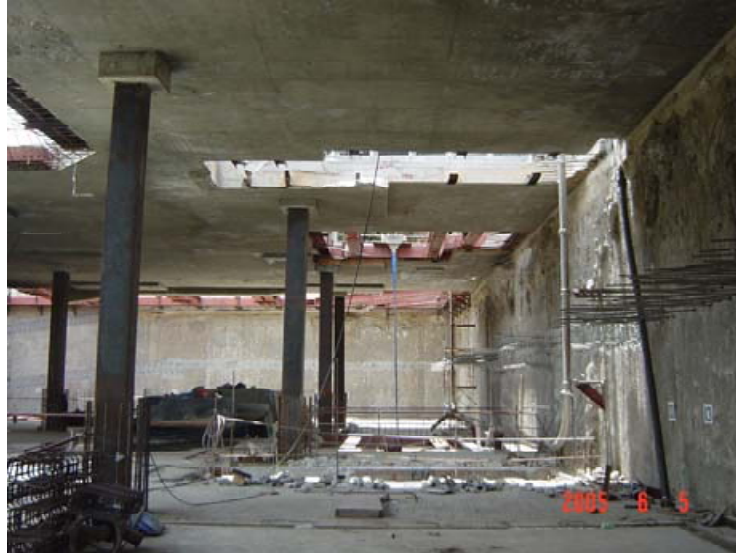
Figure 18. Photograph of D-wall after excavation
