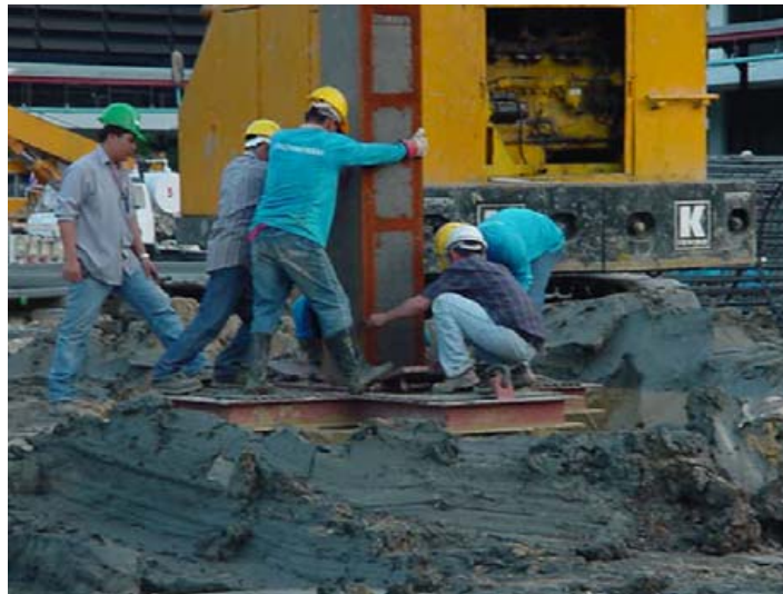
Figure 6. Photograph of stanchion installation in the bored pile
