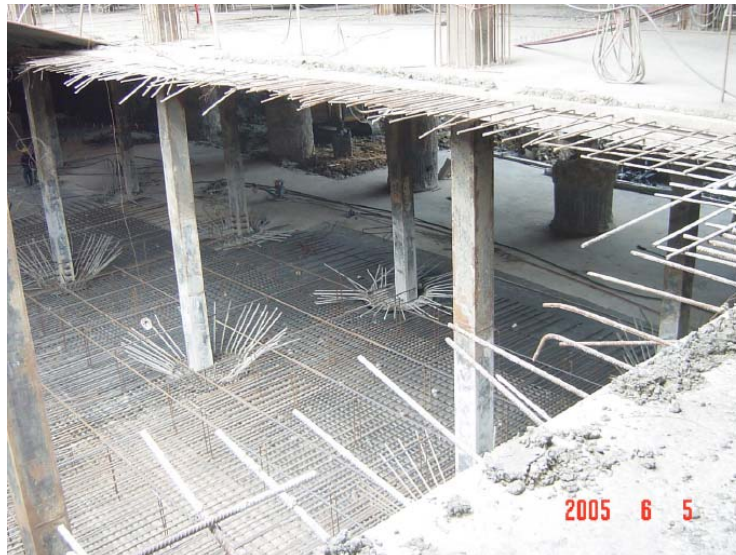
Figure 19. Photograph of base slab construction (fifth basement floor)
