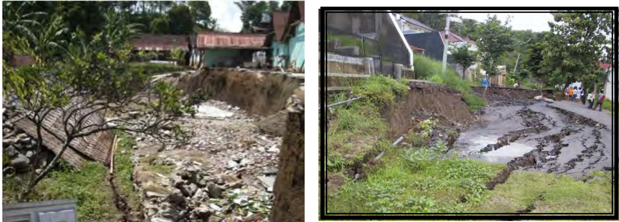
Figure 5. Subsidence induced by creep in tuffaceous silt-clay in Tengklik Village, Karanganyar Regency (left) and in Semarang, Central Java
