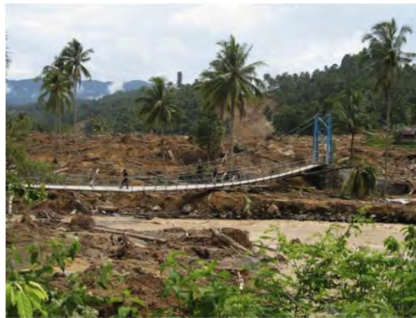
Figure 4a. Rock Slide (top) induced by extreme rainfall and earthquake of 7.6 M at Tandikat Village, Padang Pariaman Regency, West Sumatera on September 30, 2009 which continuously developed as the earth flows (bottom) and resulted in two villages and more than 100 people buried
