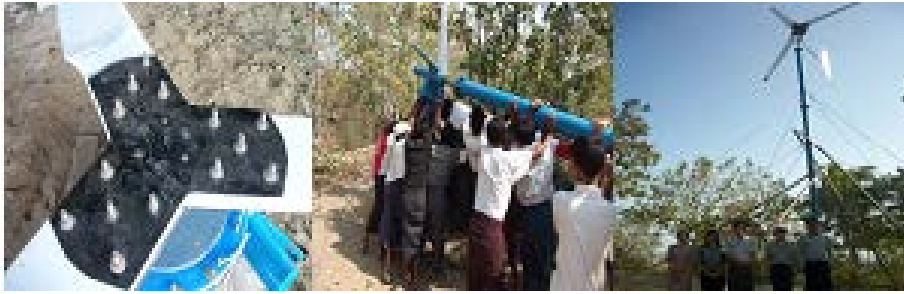
Figure 7. Preparation to raise the wind turbine
