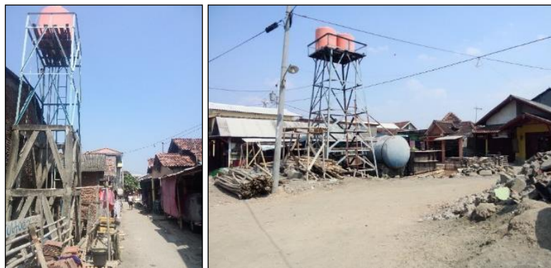
Figure 7. Water infrastructure condition in the study area (Source: Field visit, August 2015)
