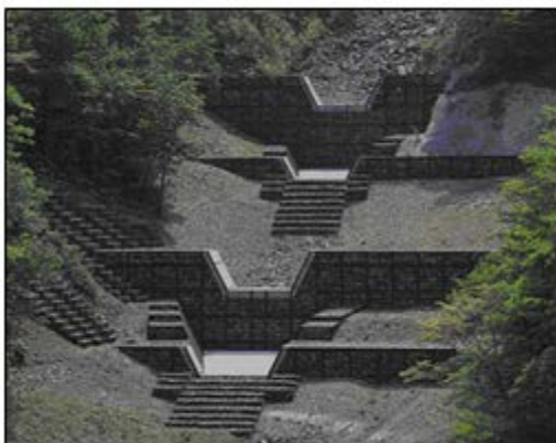
Photo 7. Steel frame dam [6]
