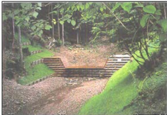
Photo 2. Wooden check dam
