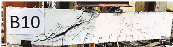
Figure 8: Cracks and failure mode of a beam with (1.5%PVA+0.375%PP), without Stirrups [55].
