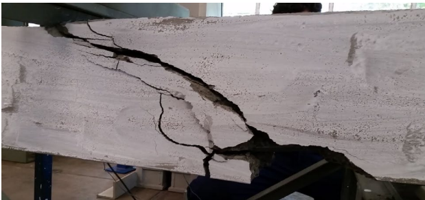
Figure 2: Shear Failure of a Reinforced Concrete beam near the prop
