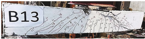
Figure 7: Cracks and failure mode of a beam with (0.75%PVA+0.75% PP) +Stirrups [55]
