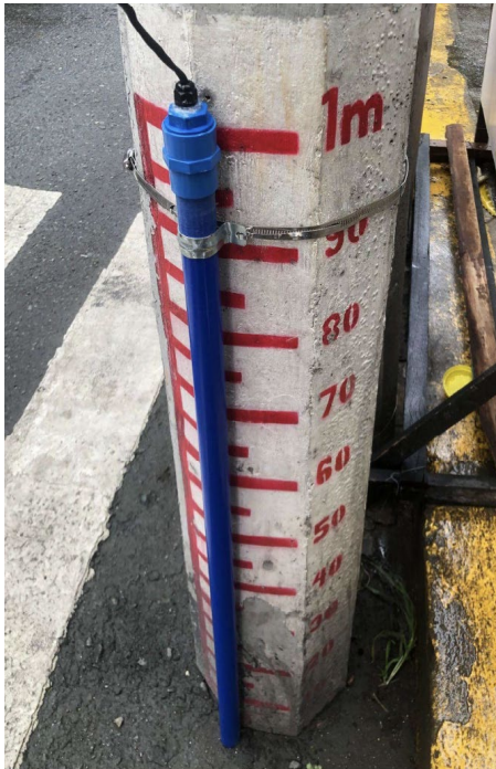
Figure 7. PVC pipe and pressure sensor setup
