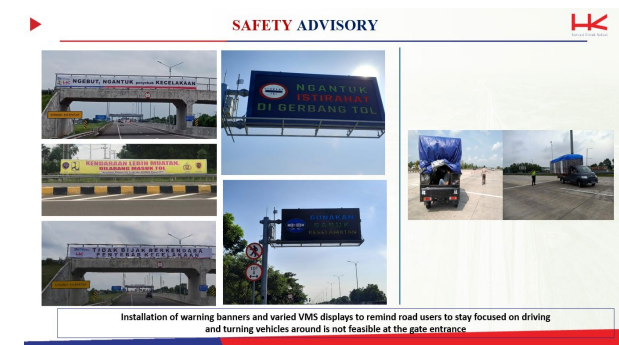
Figure 2 Barriers and VMS on Palembang-Indralaya Toll Road Source: PT Hutama Karya
