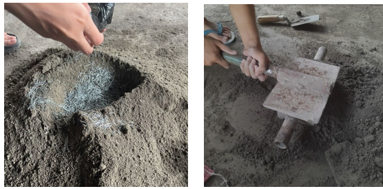
Figure 2 Paving Block Production
