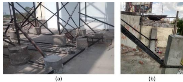
Figure 7 Billboard connections on the structure
