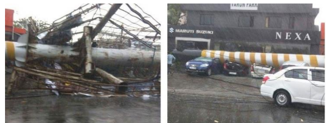
Figure 4 Damage of Billboard and partial damage of building (Jubilee Hills check post, Hyderabad, 20 May 2016)
