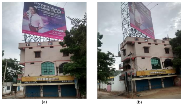
Figure 6 Existing structure considered for this study
