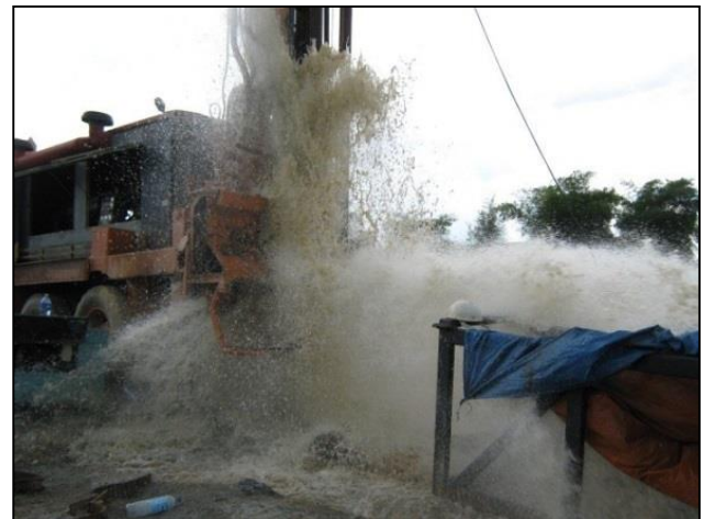
Figure 14 Water comes out during the well drilling process
