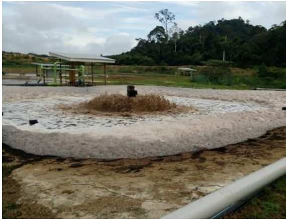
Figure 2 Scattering wastewater/sludge of surface aerator
