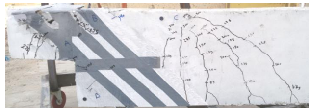
Figure 19 Cracks patterns for strengthening beams HSTR1-B
