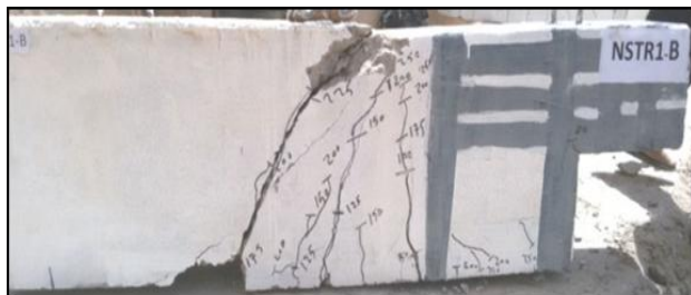
Figure 25 Cracks patterns for strengthening beams NSTR1-B
