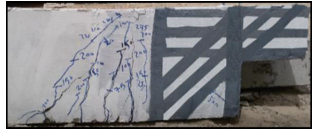
Figure 26 Cracks patterns for strengthening beams NSTR2-B
