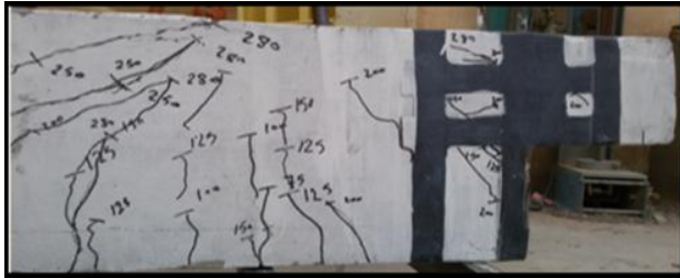
Figure 17 Cracks patterns for strengthening beams HSTR2-A
