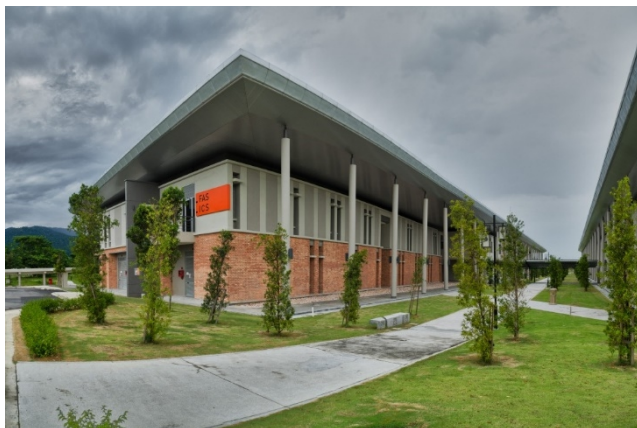
Figure 2 Prototype full scale building model located in Block N, Universiti Tunku Abdul Rahman, Perak, Malaysia
