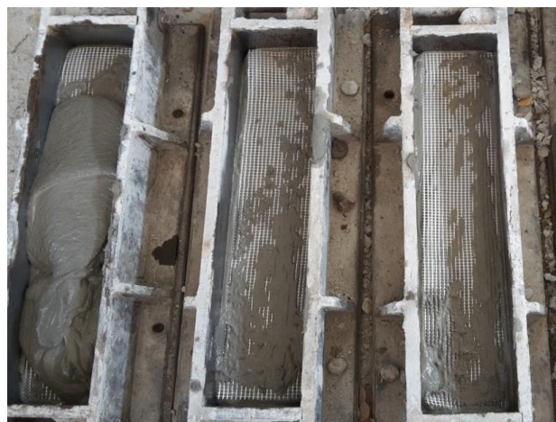
Figure 2 Fibreglass netting was placed in the moulds
