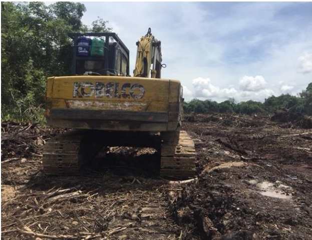
Figure 1 The use of excavator for land clearing and the preparation of oil palm plantation site in Sibul, Sarawak, Malaysia
