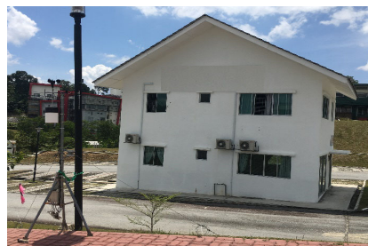
Figure 1 The double-storey detached house used in the study
