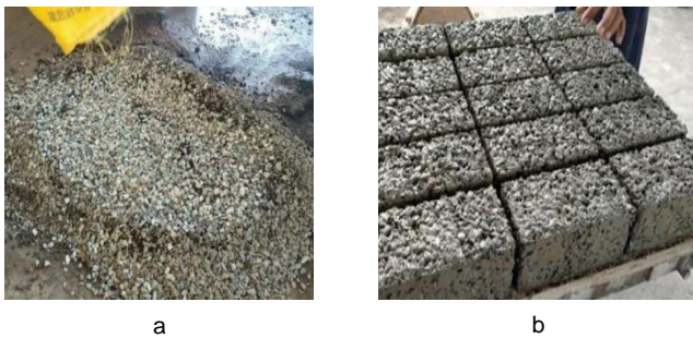
Figure 4 (a) Combining PET aggregate into porous concrete block mixtures and (b) Porous concrete block after casting
