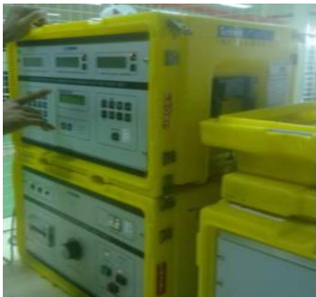
Figure 4 Equipment for dissipation factor measurement
