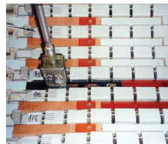
Figure 2 Typical SSC installations 5
