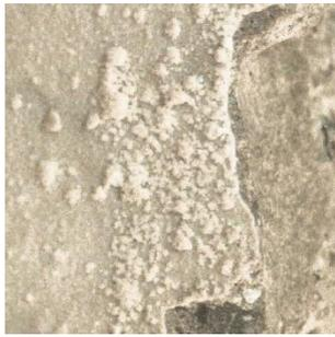
Figure 7 Efflorescence appearance on surface
