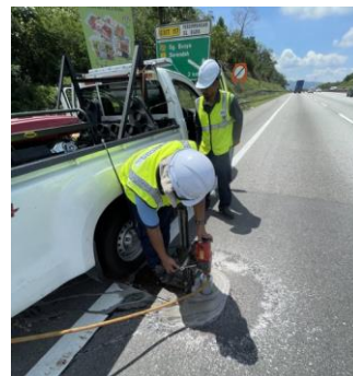
Figure 5 Coring Works in Progress
