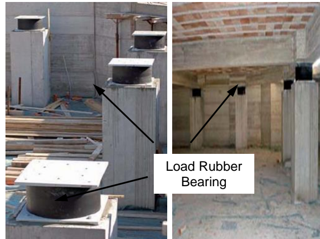
Figure 1 View of used LRB in all columns
