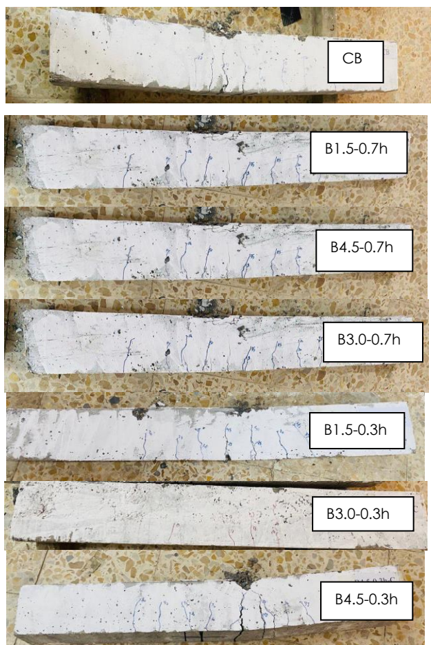
Figure 8 Crack patterns of all beams
