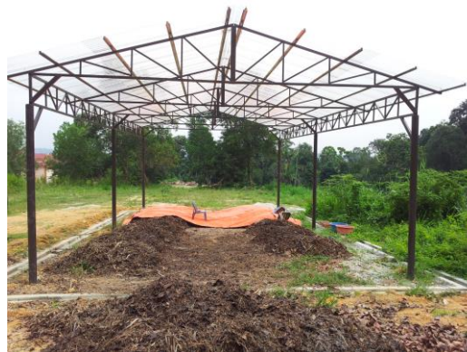
Figure 6 Pilot plant of windrow composting
