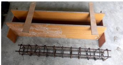
Figure 8 Preparation of Beam Reinforcement
