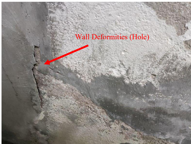
Figure 17 Uneven wall picture
