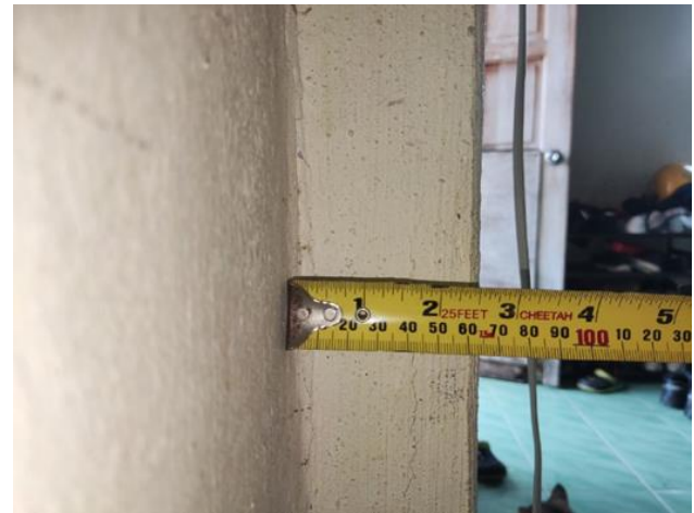
Figure 15 Measurement of Fixed Wall Depth.
