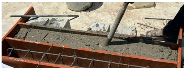
Figure 4 Pouring concrete beams
