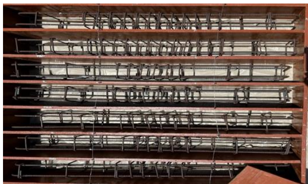
Figure 3 The formwork and reinforcement for the beams
