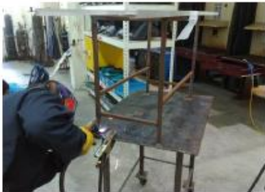
(a): Steel welding
