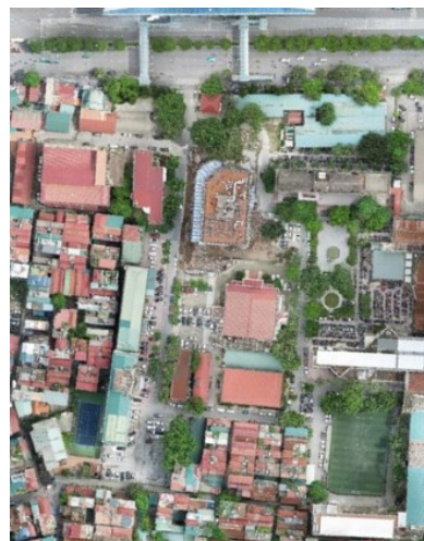
Figure 7 UAV images processed using the Matrice 350 RTK device
