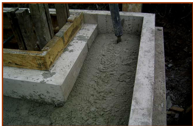
Figure 3 Utilization of lightweight foamed concrete as sewer fill in United Kingdom
