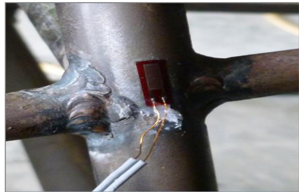
Figure 16 Strain gauge mounted on the chassis
