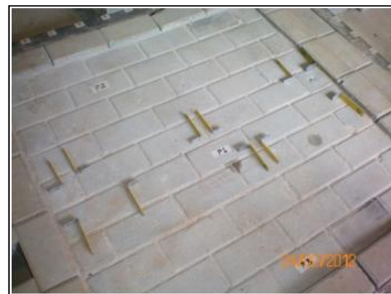
Figure 3 Eleven points were marked for horizontal loading test.
