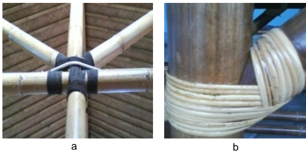
Figure 1 Connection with (a) ijuk rope and; (b) Rattan rope in bamboo truss structure. (Source: Fieldwork 2011)
