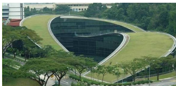
Figure 1 Extensive green roof
