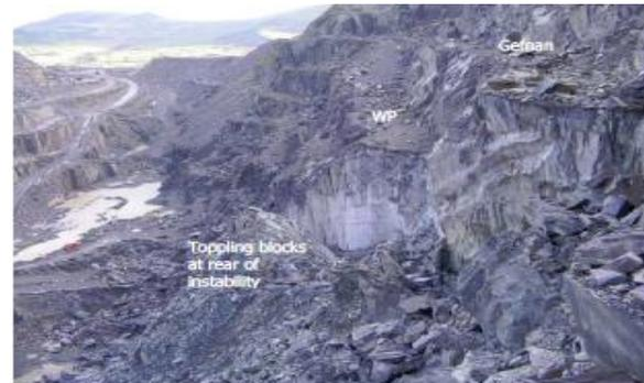
Figure 4 Flexural toppling and overturning at rear of failure
