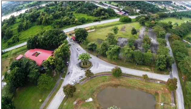
Figure 7a Traffic condition at entrance B
