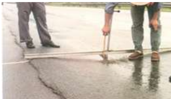
Figure 3 Rutting deformation [3]
