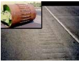
Figure 1 Shoulder rumble strips [15]
