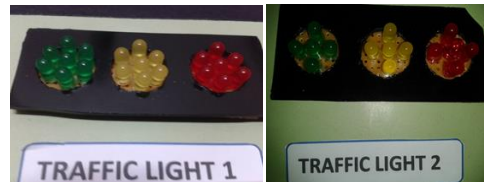
Figure 4 LED installation of traffic light
