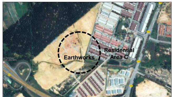
d) Taman Kempas Utama (earthworks)
