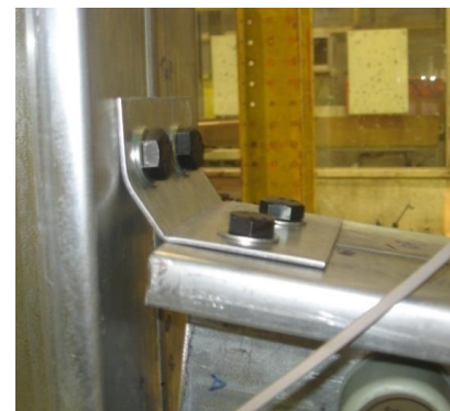
Figure 6 Failure mode for 2 mm thickness of flange cleat which is flange cleat in bending
