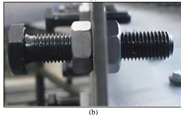
**Figure 1** The shear connectors used, (a) Types of shear connection; (b) Method of nuts fastening
