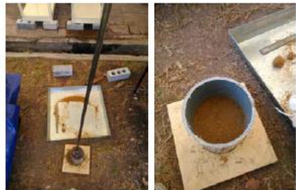
Figure 3 Throughout the process of compacting soil-cement mixture in the PVC cylinder
