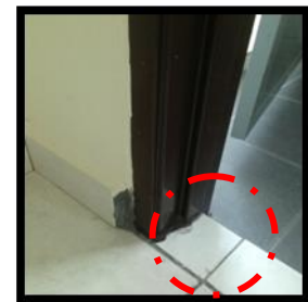
Figure 2 Floor finishes are not closely
