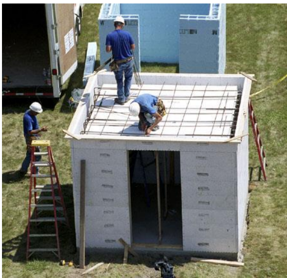
Figure 1 FEMA safe room construction [7]
