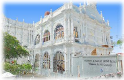
Figure 6 3D point cloud data of Penang Museum
