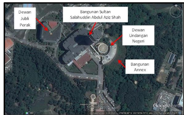
Figure 1 Selangor state secretary complex satellite view.
