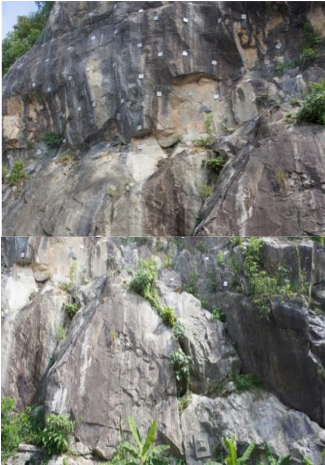
Figure 4 Wire mesh and rock bolt installed on site
